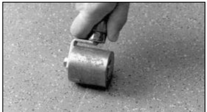
Figure 7. Hand-roll the seam area gently with a hand roller to smooth seam.
