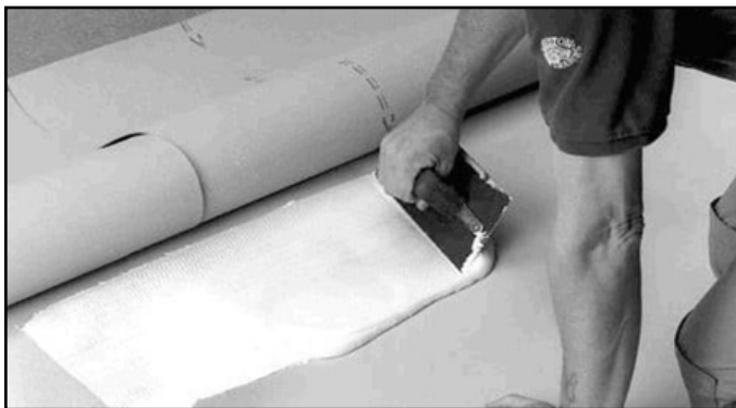
Figure 5. Spreading Adhesive.
