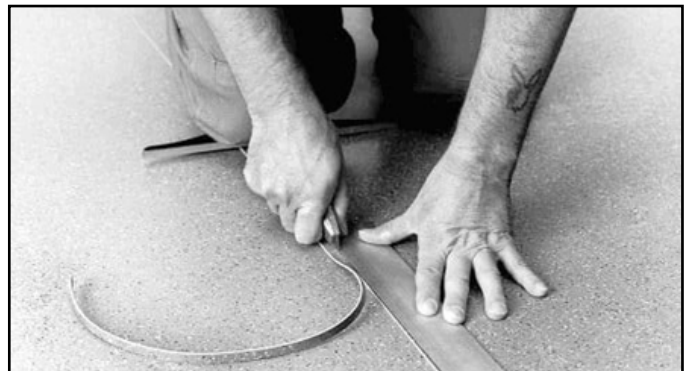
Figure 4. Cutting the Seam.
