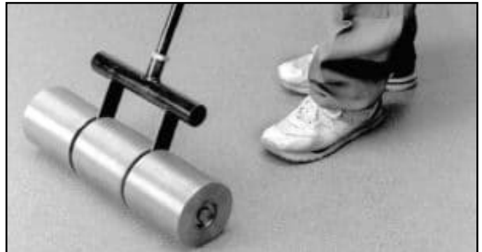
Figure 6. Roller to firmly embed the tiles/rolls into the adhesive.
