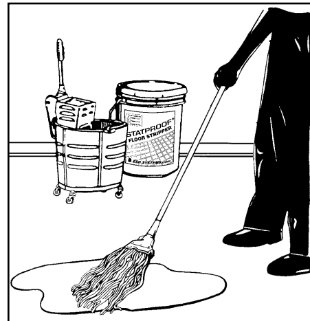
Figure 3. Applying stripper.
